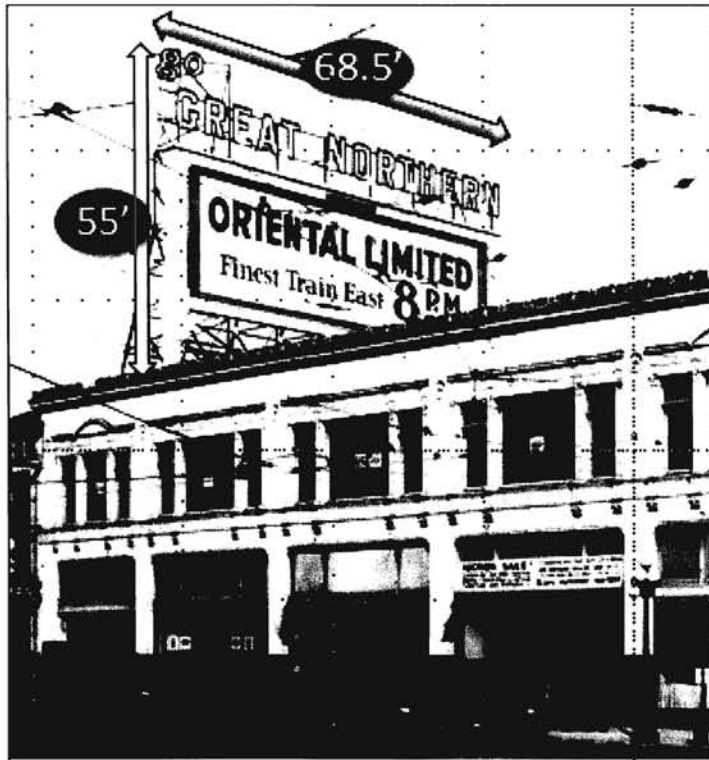
Historical Photograph of Sign with Great Northern Copy. R 00575. Dimensions from 1941 permit superimposed onto image.
