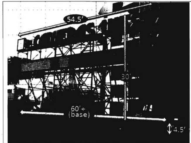
Sign with Cameras West Copy Before Repairs. R 00751. Measurements superimposed onto image.
